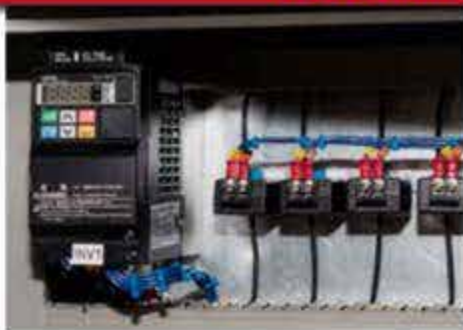
An Omron MX2 inverter in a Starview packaging machine.
